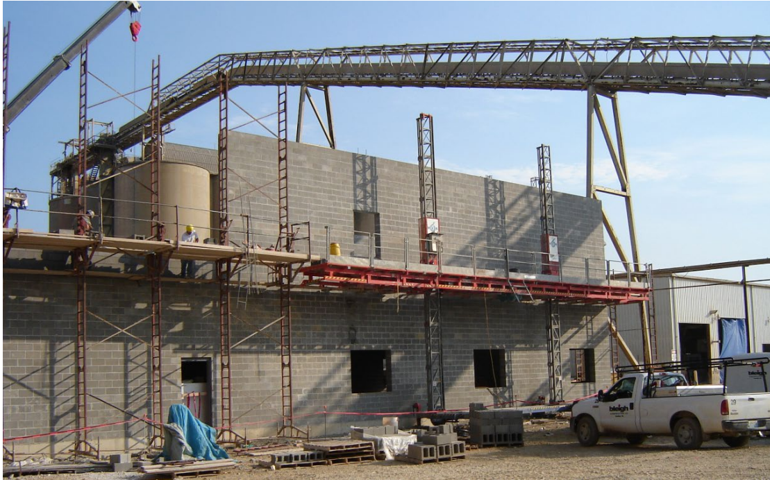
Figure 10: Elevating Scaffold keep the Masons at ideal working elevation
