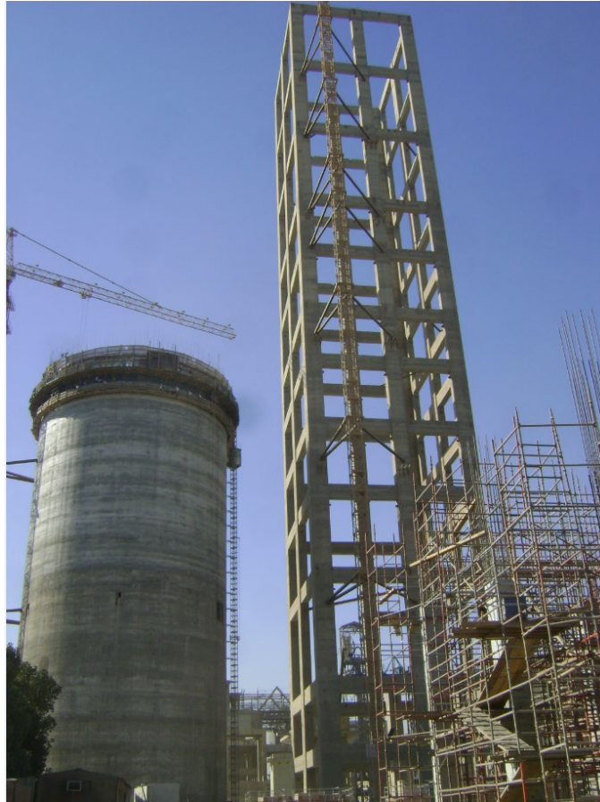
Figure 4, Project 2 - Slip forming the homo silo and pre-heater structure
