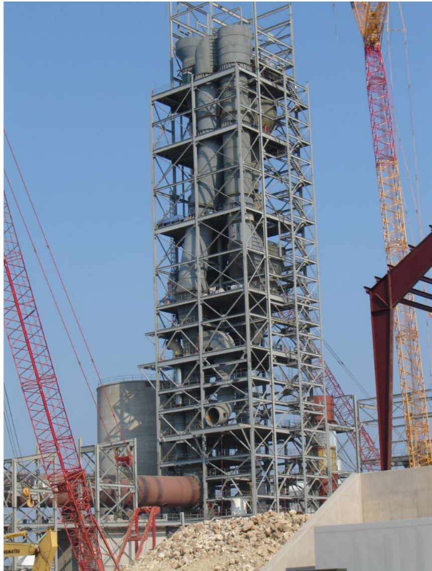
Figure 5, Project 1 - during the pre-heater construction
