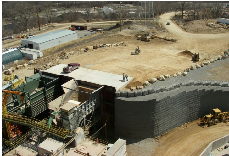
Figure 12; Project 1 - Contractor used rock gabions for retaining walls
