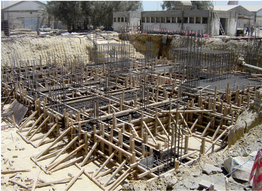
Figure 8, Project 2 - Pre-heater foundation formwork
