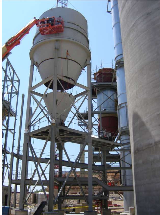
Figure 9, Project 1 - A very minimal amount of scaffold was used. Man lifts are very prevalent.
