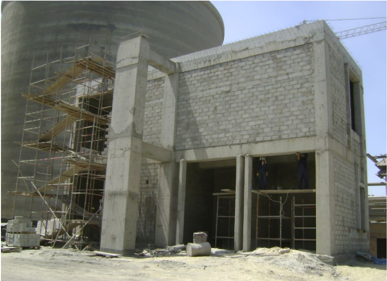
Figure 11, Project 2 - Masonry Scaffold with Ramps for efficient work height
