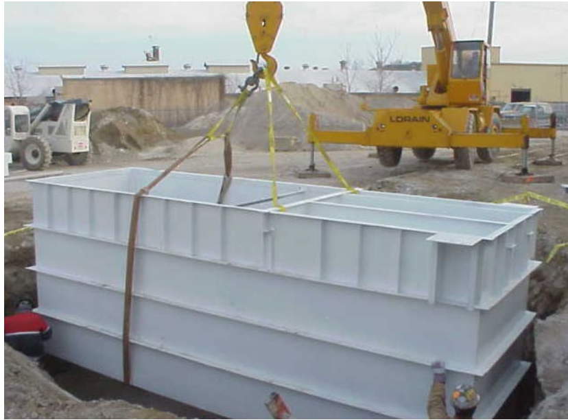
Figure 2; Direct Burial Pit Form
