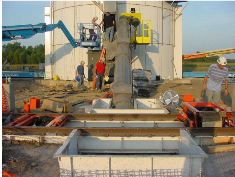
Figure 4: Two Position Hopper-car Unloading pit (cement)
