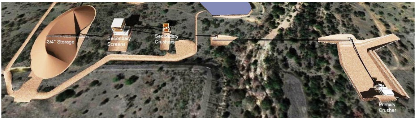
Figure 3: View from the back of the property. The primary crusher is on the right
