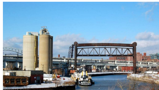
Figure 5: Cement Silo Storage with Truck and Rail Disbursing (photo courtesy of boatnerd.com)
