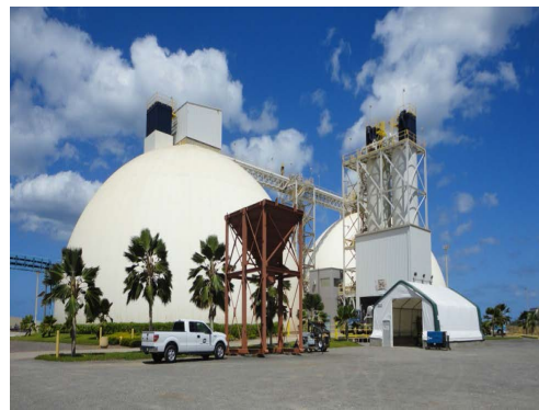
Figure 4: Typical Cement Dome Storage, (photo courtesy of HDOT)
