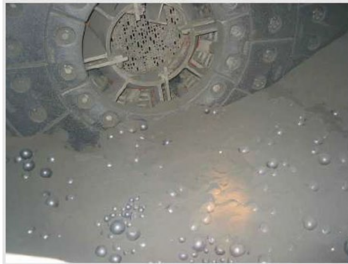
Condition in one of the grinding chambers of the mill
